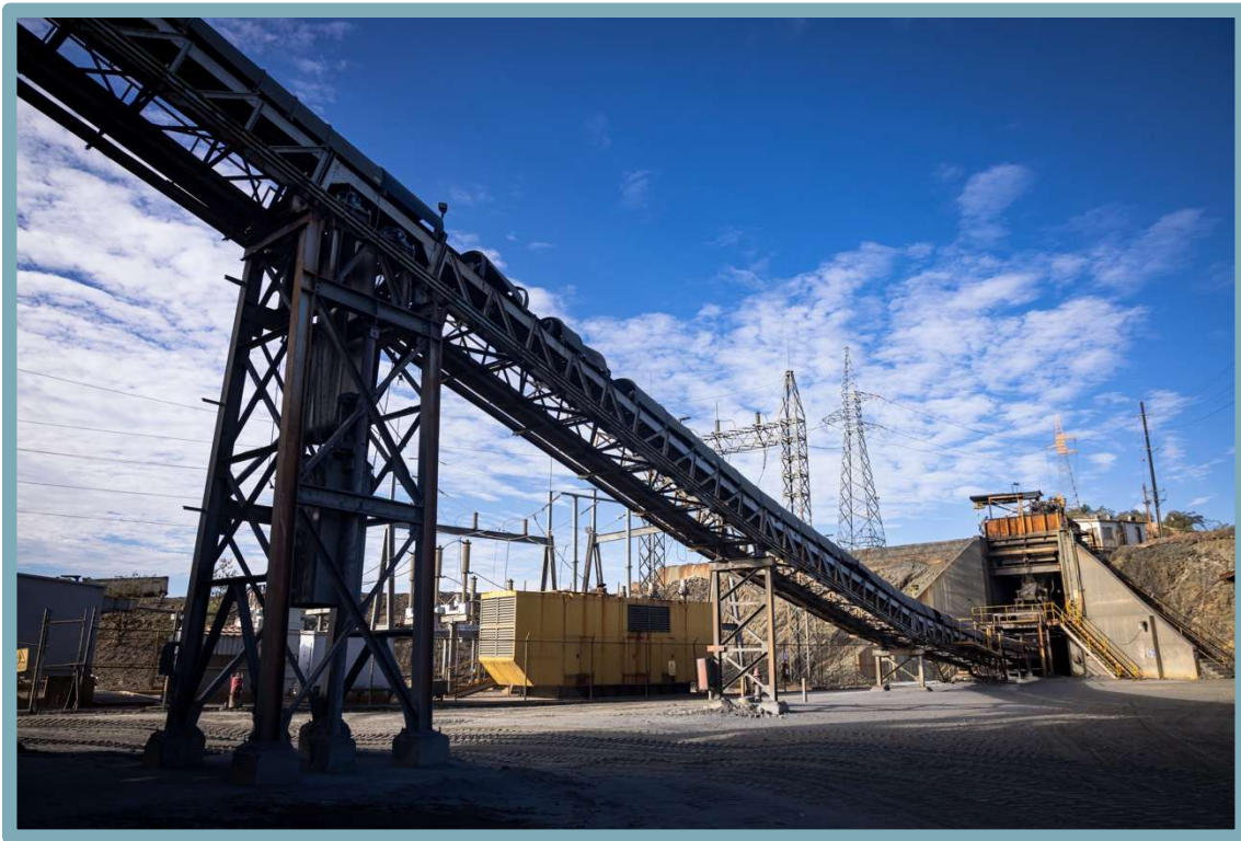
Conveyor at Campo Morado plant
