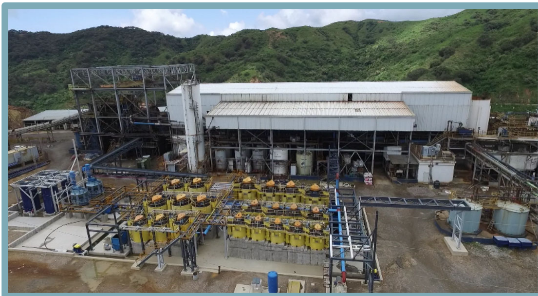
Flotation Circuit and Plant at Campo Morado
