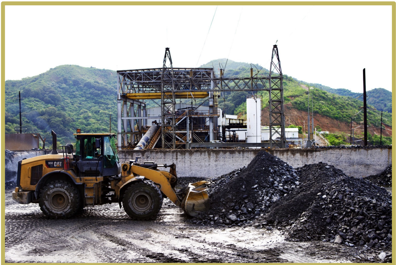
Feeding Secondary Crusher at Campo Morado
