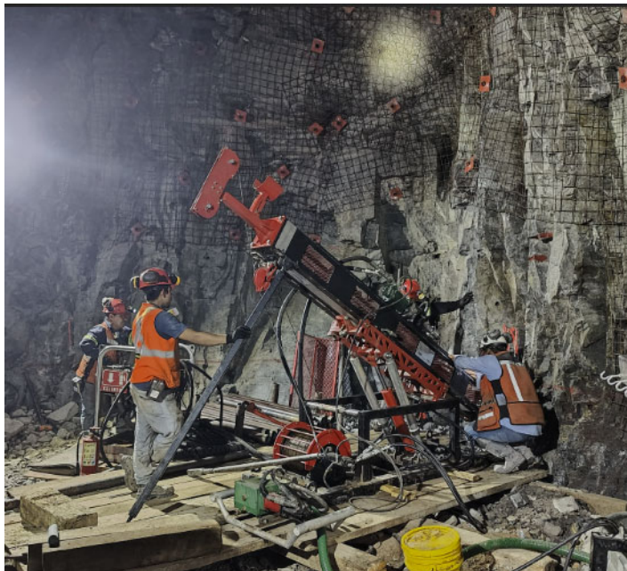
Underground drilling at Tahuehueto
