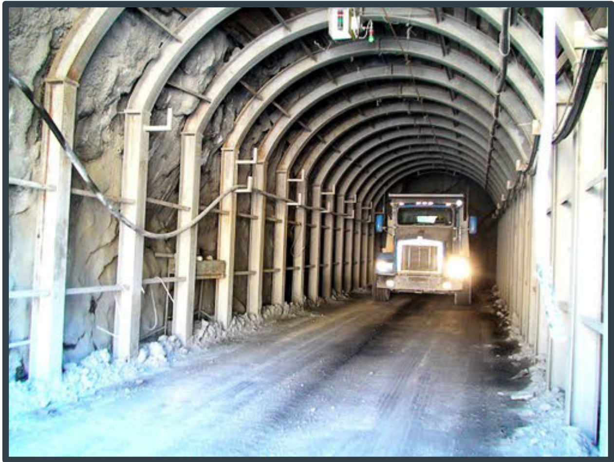
Underground Mine Entrance at Campo Morado
