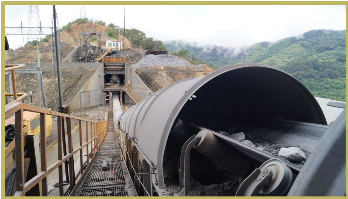
Crushed ore on conveyor belt at Campo Morado
