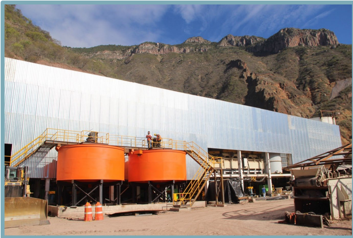
Milling, flotation and concentrate filtration building at Tahuehueto
