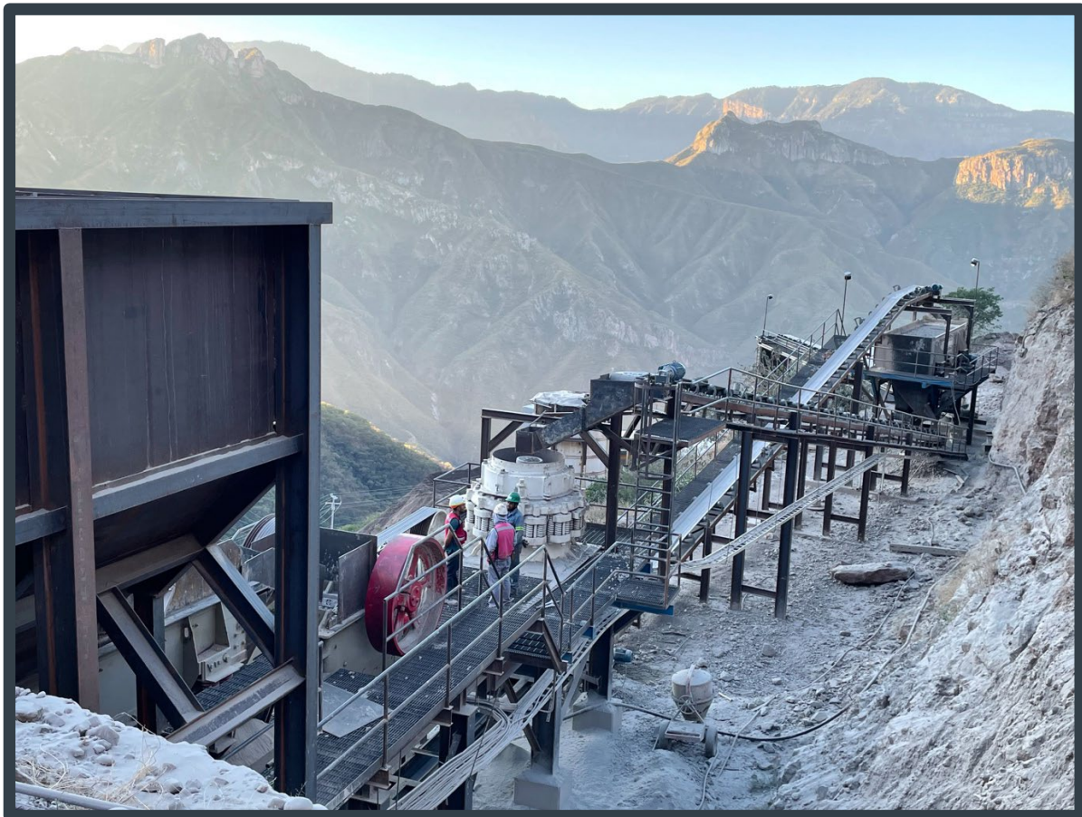
Tahuehueto crushing circuit under construction
