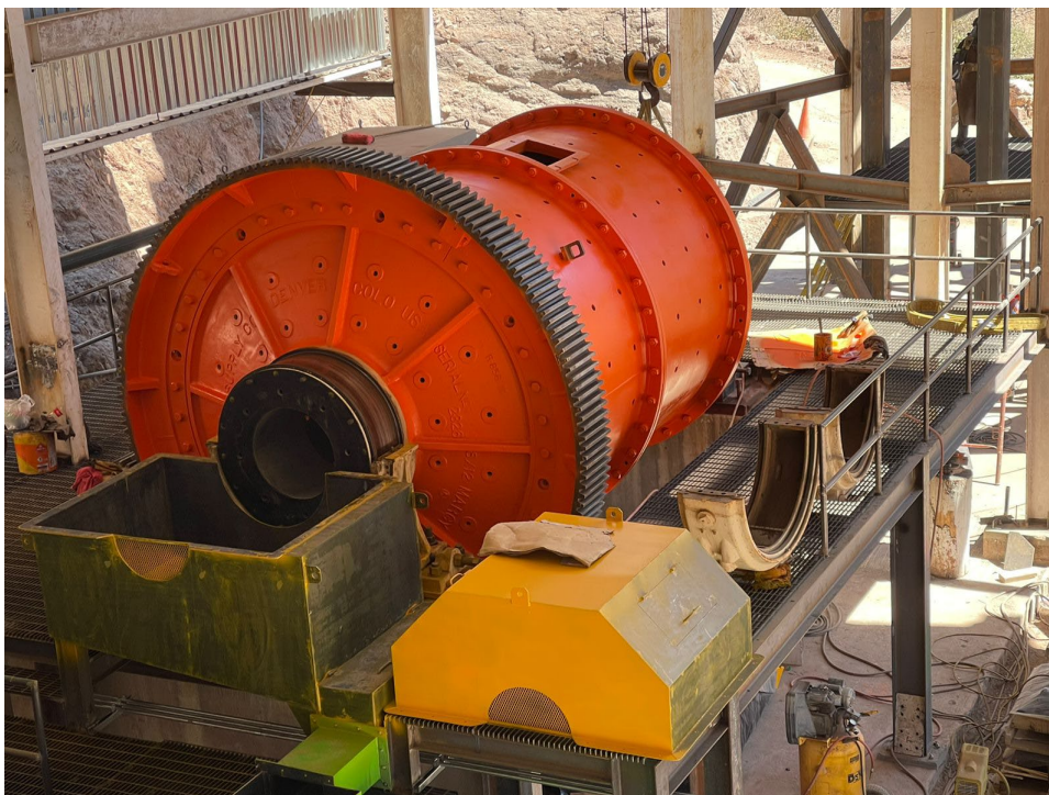
1 st Ball Mill Being Installed
