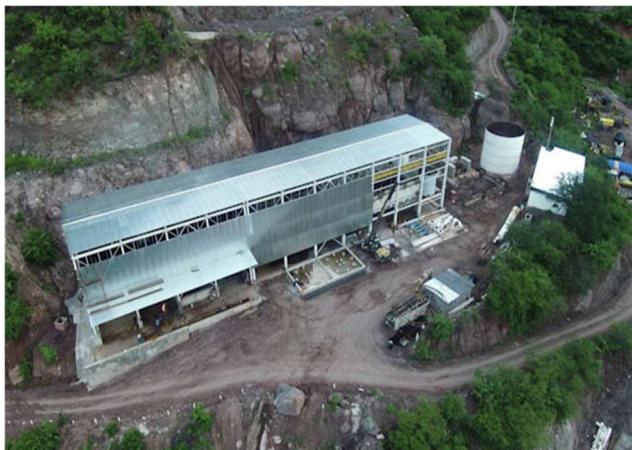
Aerial View of Milling Facility
