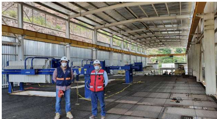
Mill Concentrate Filtration Area
