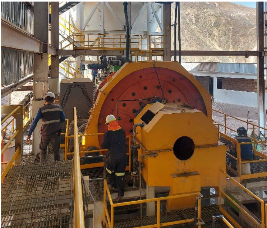
1 st Ball Mill Being Installed
