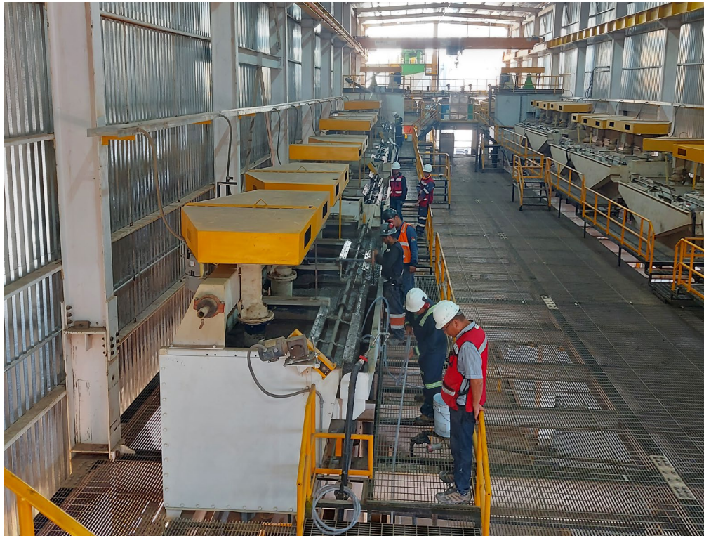
Mill Concentrate Filtration Area
