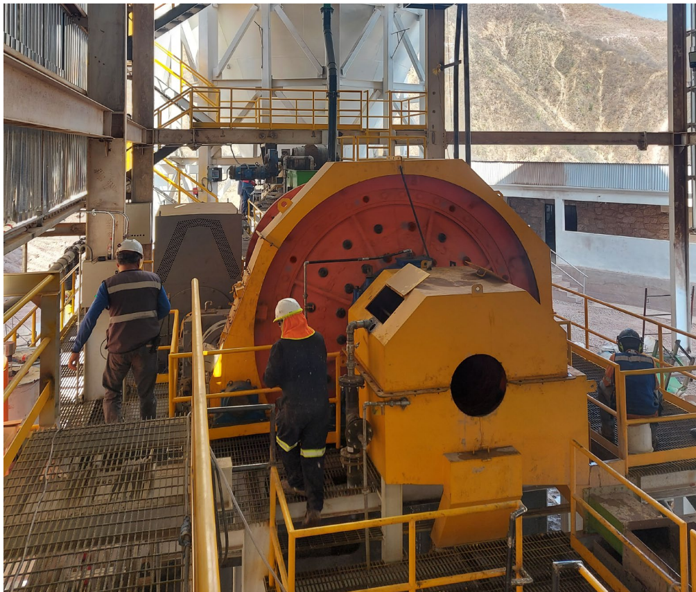
1 st Ball Mill Being Installed
