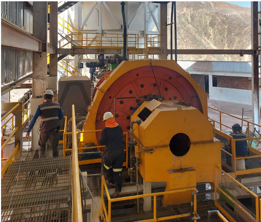
1 st Ball Mill Being Installed
