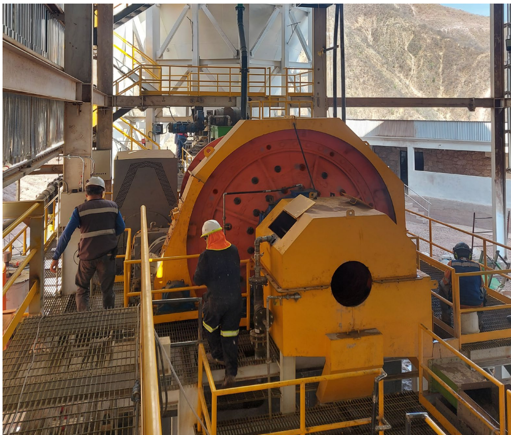
1 st Ball Mill Being Installed
