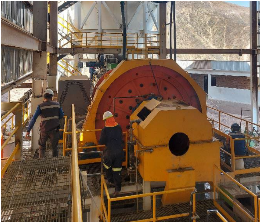
1 st Ball Mill Being Installed
